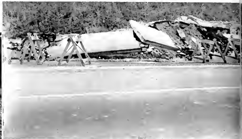
These pictures show volume and force developed by a circular type slide, such as occurred at Kellogg Hills
